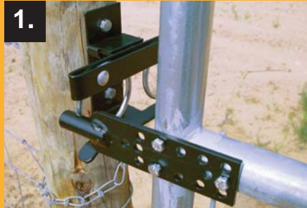
1. The gate swings closed and the striker bar hits the ring.
